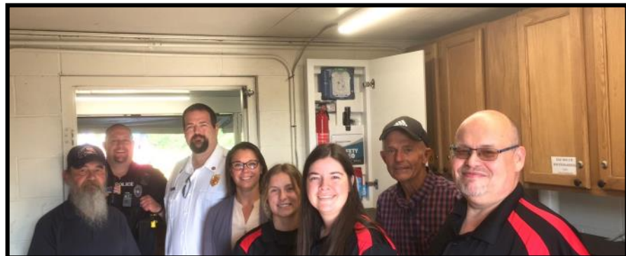
New Defibrillator installation at the Village Park
